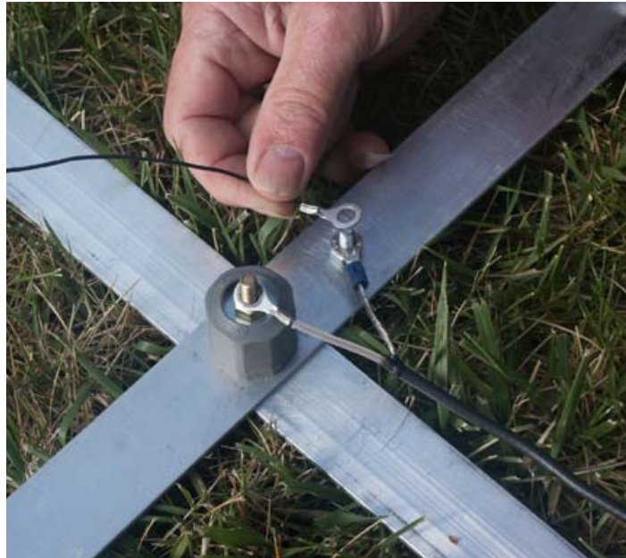
Figure 3: Installing Radial Wires
