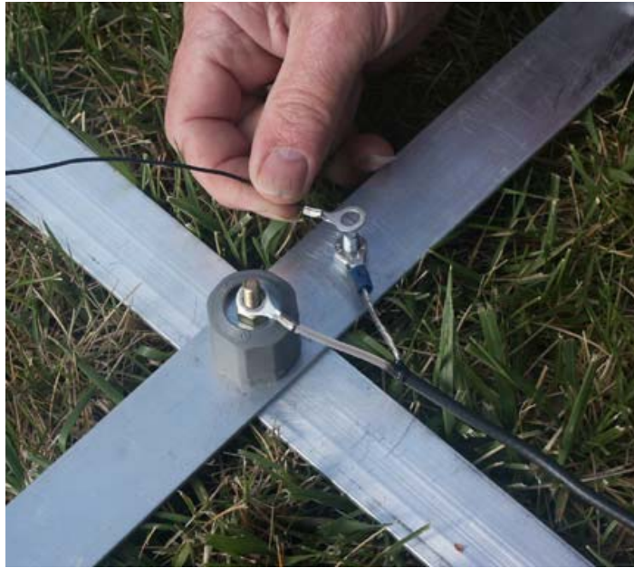
Figure 3: Installing Radial Wires
