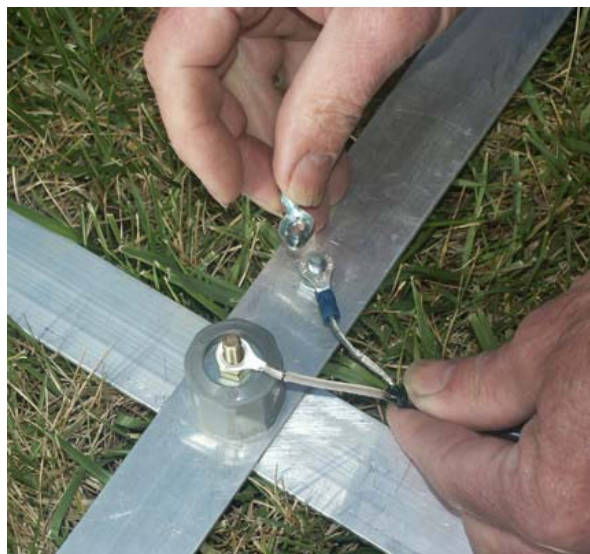
Figure 2: Install Coaxial Pigtail
