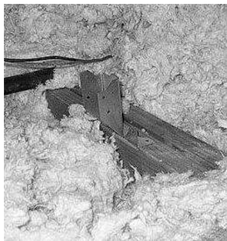
Nail the bracket to a rafter
